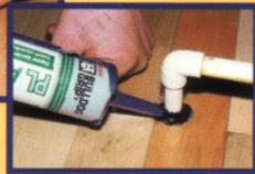
Use an acoustic sealer to fill the 3/8" (9 mm) space completely up to the covering. Do the same thing for any obstacles.
